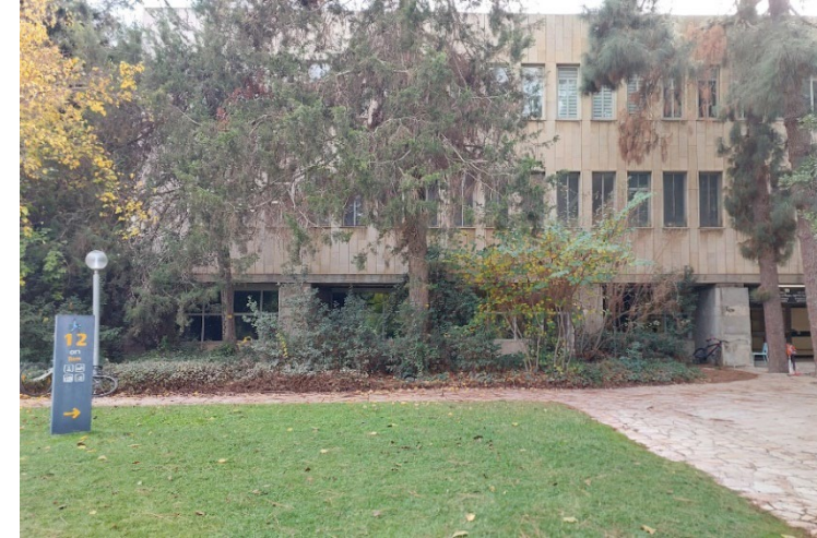
Old CS Building
